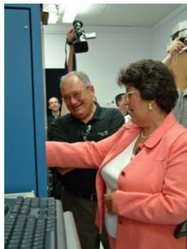
Commissioners patch in a high-speed fiber on July 18.
