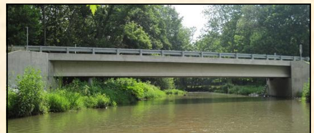
Murkle Road over Big Pipe Creek
