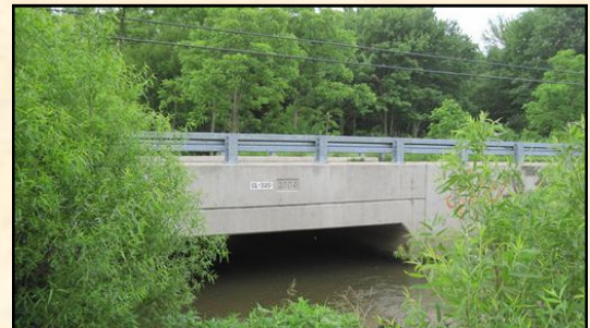
Freter Road over Piney Run
