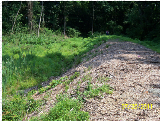
The current condition of the facility.
