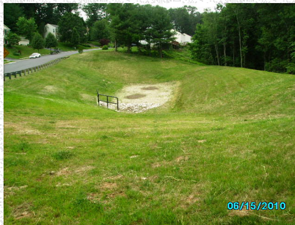
The facility has been mowed for the first time.
