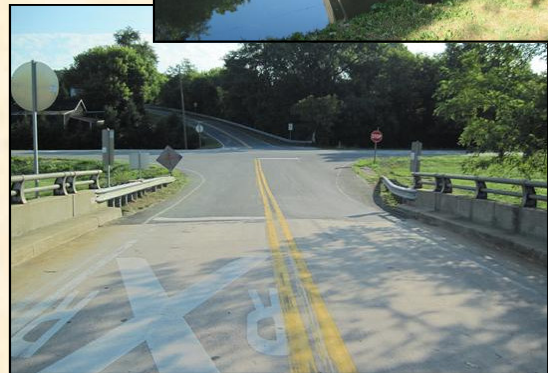
Top photo: view of Shepherds Mill Road bridge Bottom photo: looking at the approach to MD 75
