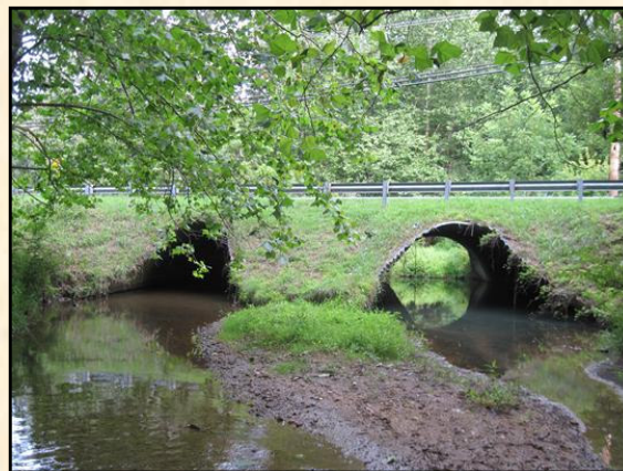
End view of the twin metal culverts on White Rock Road.
