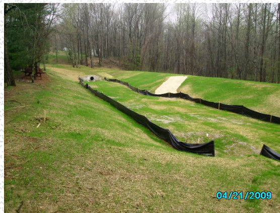
The above picture shows the facility with grass beginning to grow.
