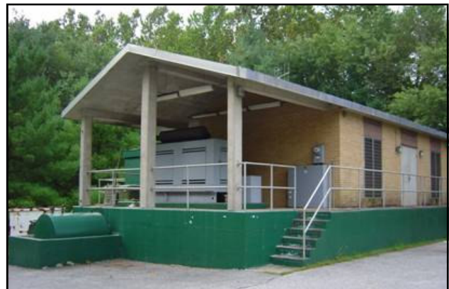
Exterior of the Piney Run pumping station, the largest in the Freedom wastewater system.
